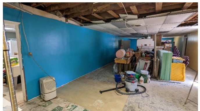
Church basement – Game room – drywall done/painted.
