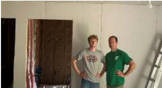
John and Zane Installing Drywall
