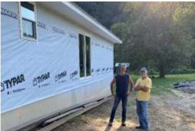
Soffit and Fascia by Vick, Jason, and John
