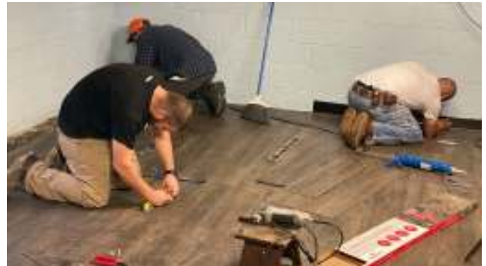
Installing New Flooring
