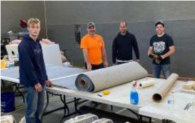
Gym Carpet Getting Installed
