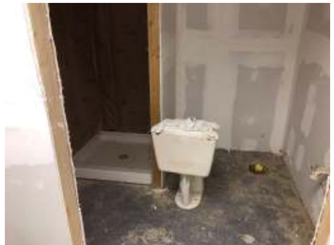
Gym Bathroom with Drywall Replaced
