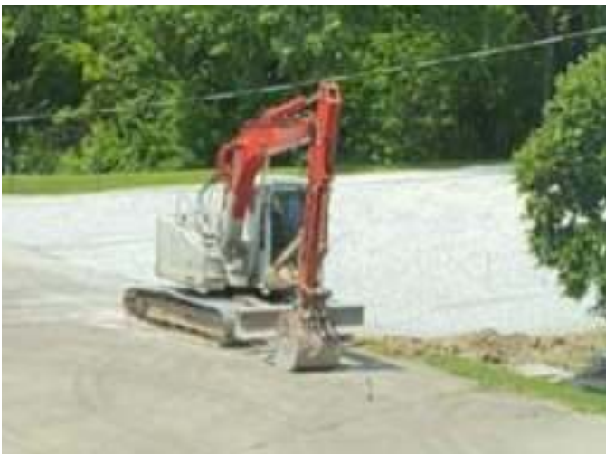
Work Finished on New Parking Lot
