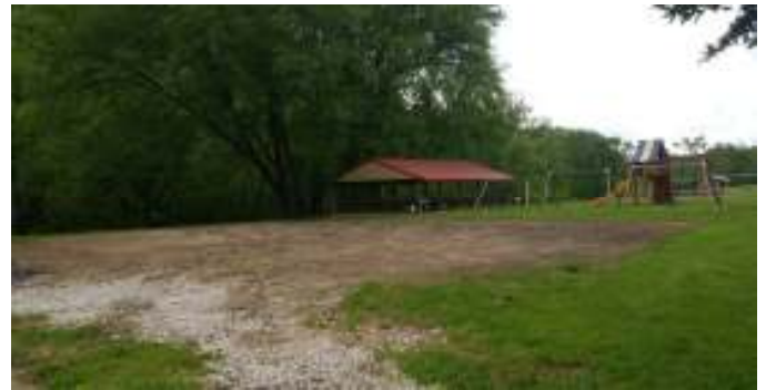
Work on New Parking Lot
