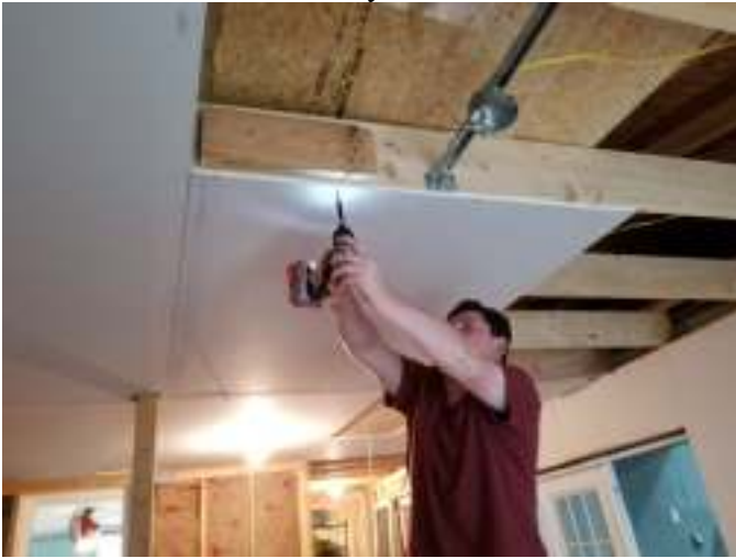
One of the Teens Hanging Drywall
