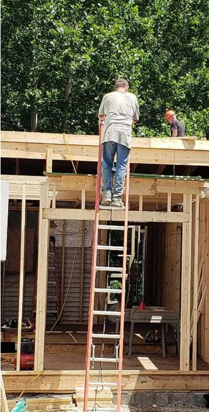
Building in Progress
