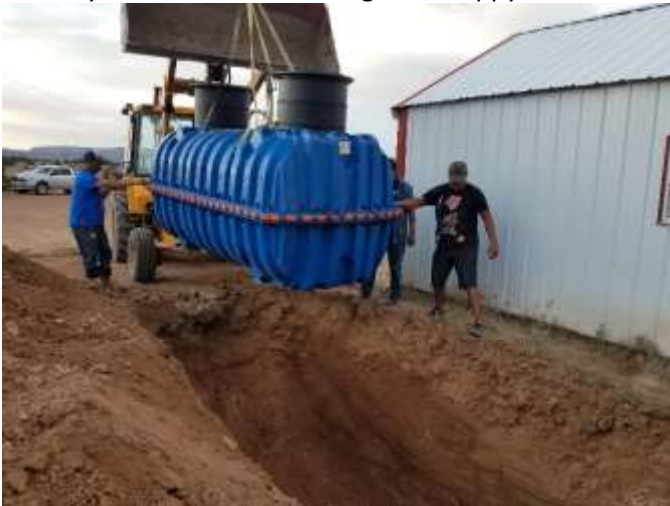
A water tank getting installed in New Mexico
